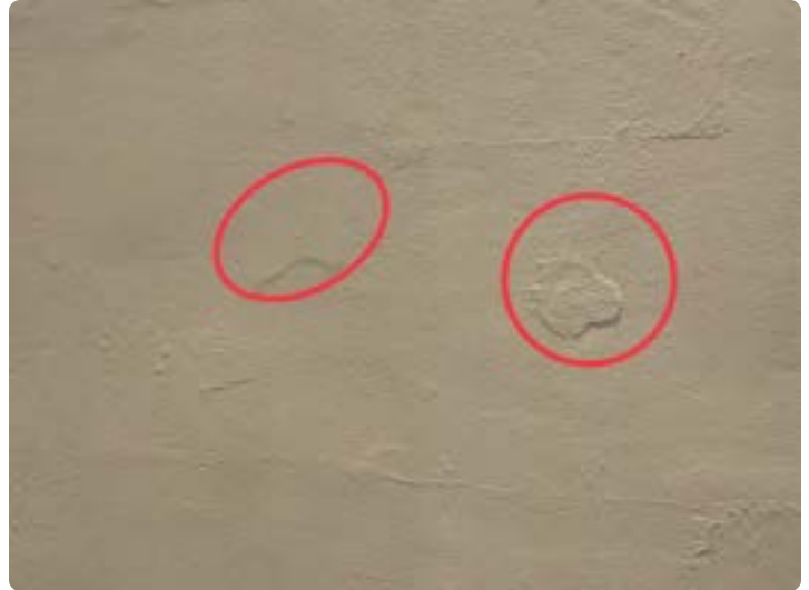
Small areas of concrete spalling on north side roof exterior stairwell wall
