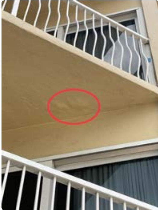
Bulges in balcony soffit on second balcony from left on the left side of the front elevation. Unclear from ground if area is due to concrete spalling, past remediation, or paint bubbling.
