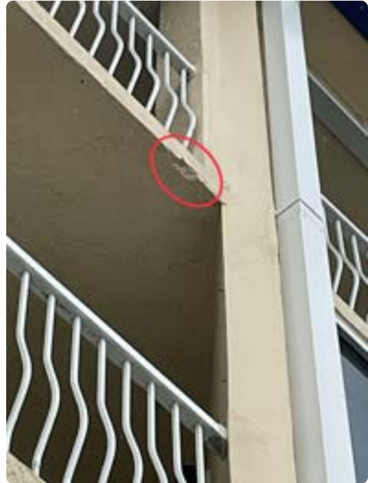
Concrete spalling on balcony slab near middle of rear elevation
