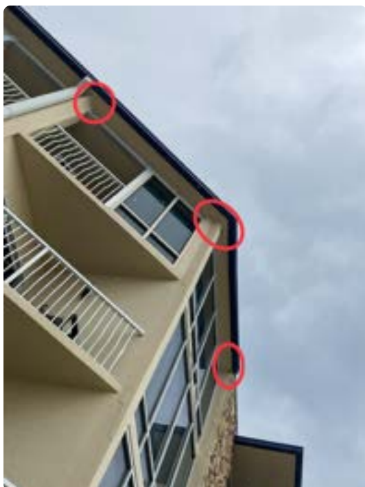
Multiple areas of concrete falling on roof soffit on right side of rear elevation
