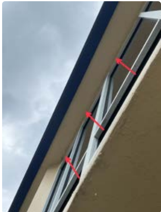
Concrete spalling in roof soffit above Unit 4022
