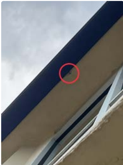
Small area of concrete spalling on roof soffit above Unit 4014
