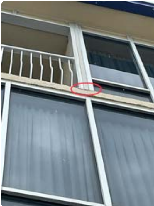
Concrete spalling at base of demising wall on balcony near blue tarp on rear elevation
