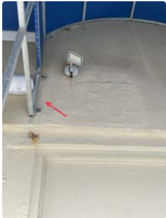
Crack around previous remediation on right elevation
