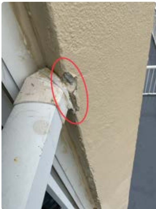
Chip in exterior wall near railing connection on Unit 2016 balcony. Area should be sealed to prevent water intrusion
