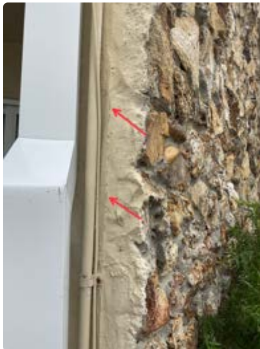
Cracks in sealant between exterior wall and stone cladding on left side of front elevation
