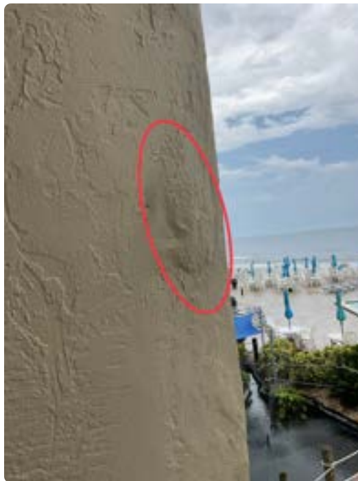
Hollow concrete behind paint bubbling on unit 2000 balcony demising wall
