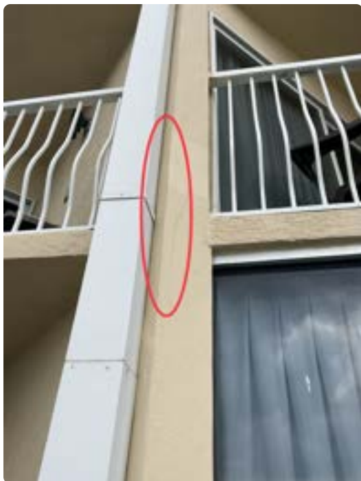
Concrete spalling on demising wall near 4th balcony from left from pool entry door
