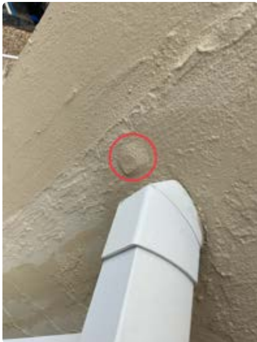
Small area of concrete spalling below railing connection on Unit 3014 balcony
