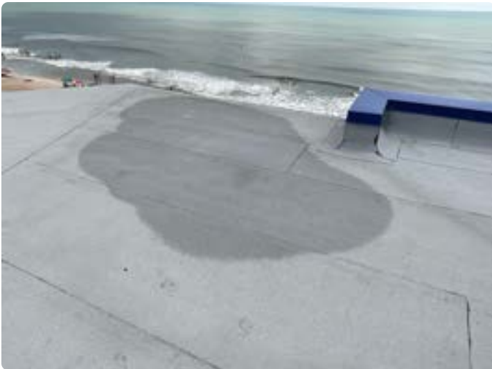
Small area of water ponding on roof
