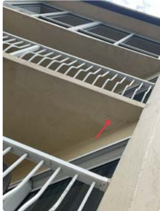
Cracks in area of previous remediation on second floor, second balcony from right on the left side of the front elevation
