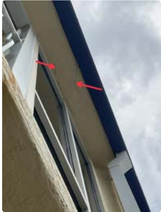
Concrete spalling in roof soffit above Unit 4005
