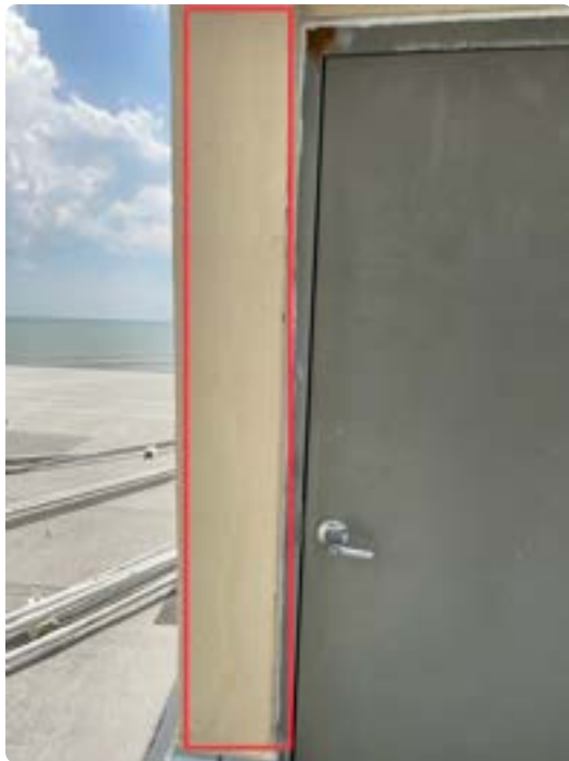
Concrete spalling on exterior wall around north side roof entry door
