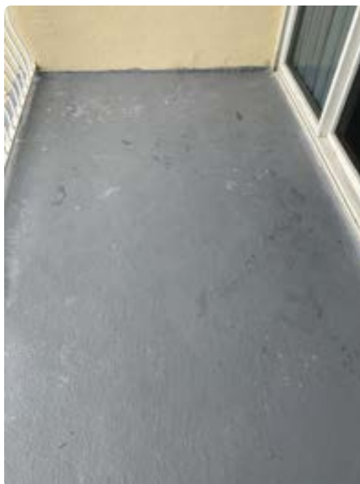
Delaminated coating on Unit 2000 balcony
