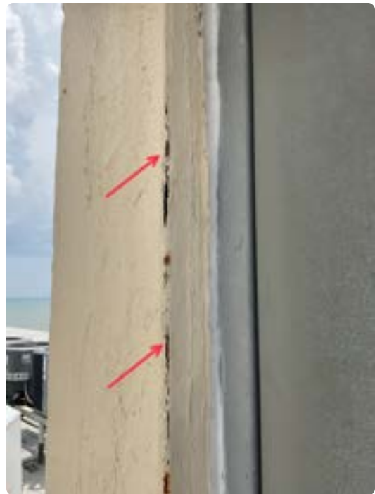
Cracks in stucco allowing for water intrusion into exterior wall near north side roof entry door
