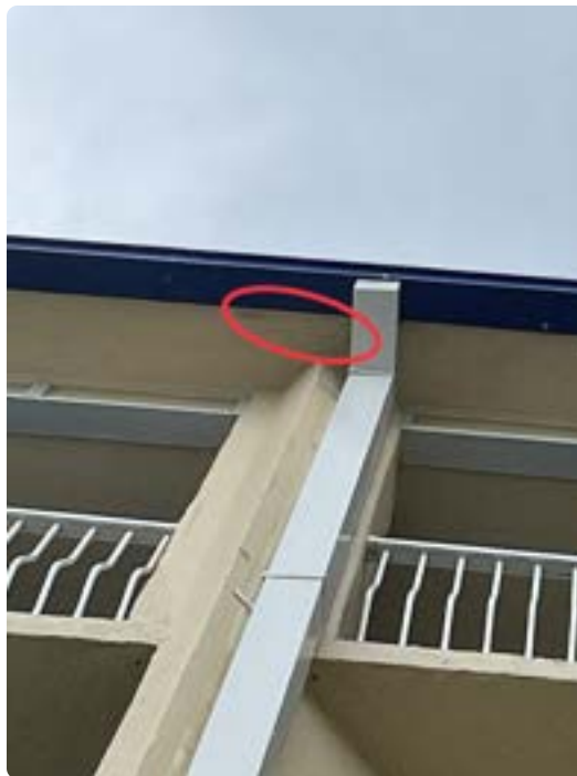
Concrete spalling on roof soffit above balcony near shed on rear elevation
