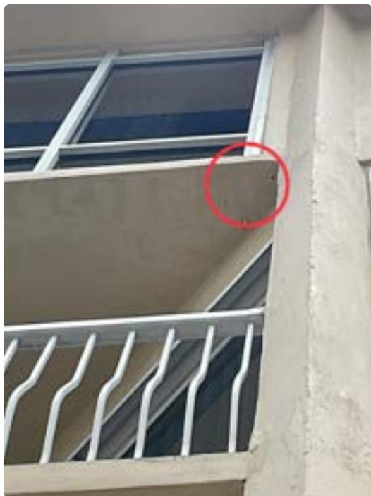
Cracks in area of previous remediation on third floor, second balcony from right on the left side of the front elevation
