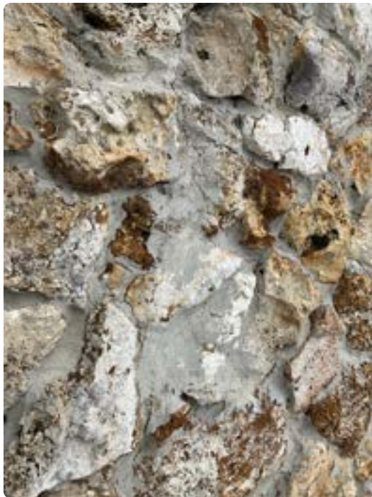
Cracks throughout grout on stone facade on left side of rear elevation
