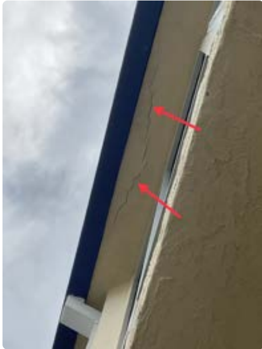
Concrete spalling on top floor soffit above Unit 4004
