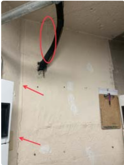
Cracking and spalling concrete on block wall in housekeeping laundry room. Entire area is hollow when sounded.
