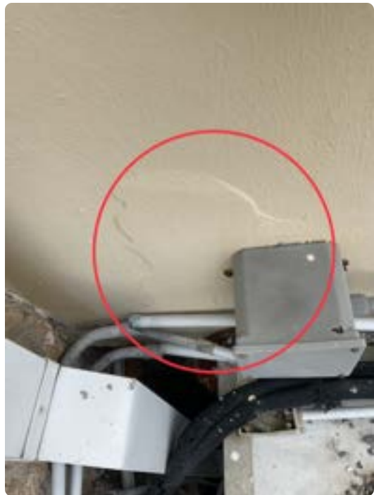
Concrete spalling on balcony wall on far-left side of rear elevation
