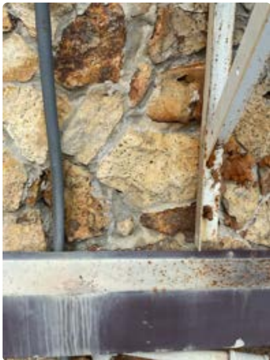
Cracks in stone facade and grout on right elevation
