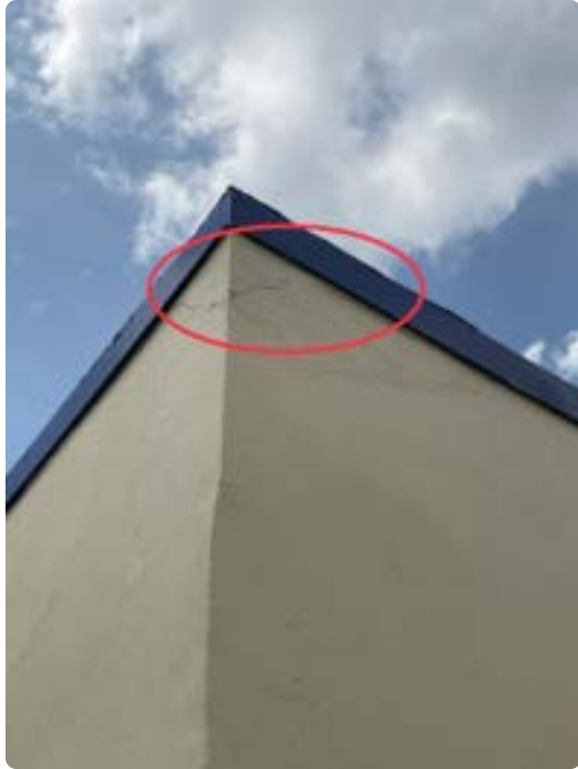
Concrete spalling at top of north side exterior stairwell wall on roof
