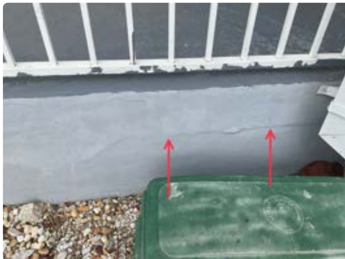
Crack in patio wall and small area of concrete spalling on far-right patio on right side of front elevation
