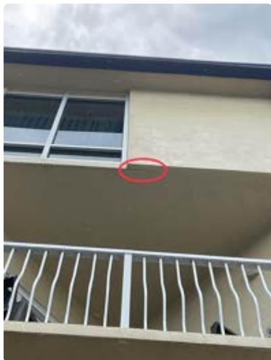
Crack in far-left balcony soffit on right side of right elevation
