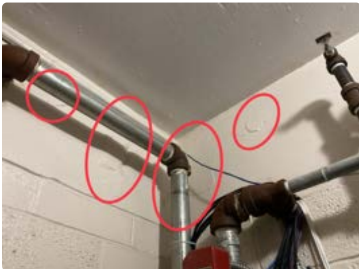
Possible concrete spalling on inside of stairwell near Unit 4003. Unclear if areas are spalling or a previous patch.
