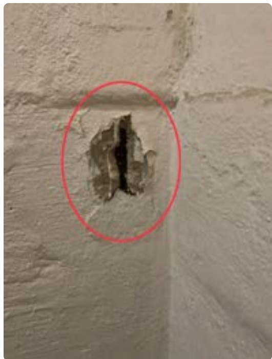
Concrete spalling with exposed corroded rebar on interior stairwell wall near Unit 4003
