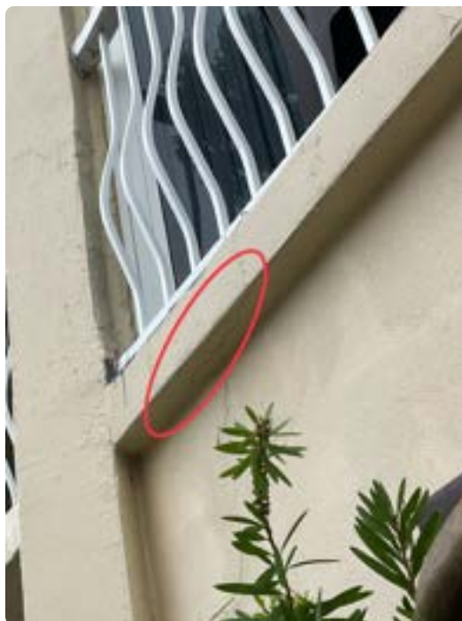
Crack below balcony slab on second floor, far-left balcony on right side of front elevation
