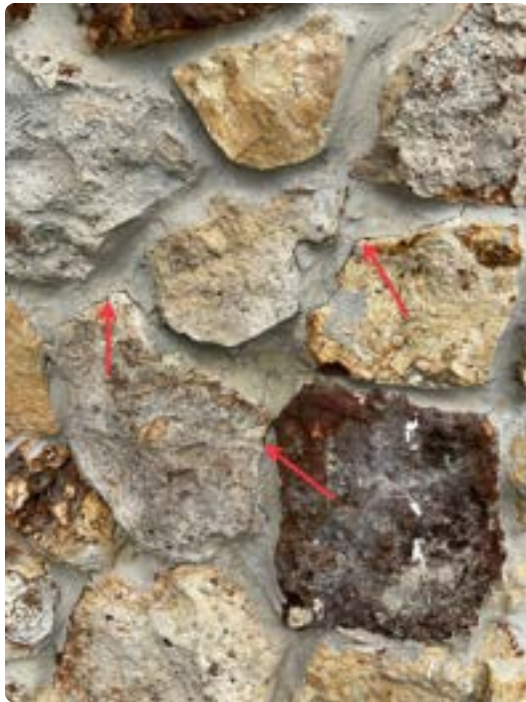
Cracks in grout around stone cladding on right side of front elevation
