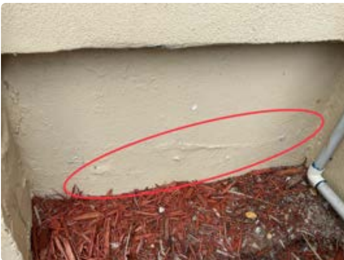
Concrete spalling at base of exterior wall near stone cladding near far-left balcony on the right side of the front elevation. Area is hollow when sounded.
