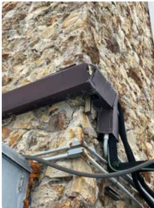
Large cracks in grout in stone facade on far-right side of right elevation
