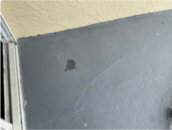
Apparent previous remediation on Unit 2004 balcony slab. Area is not hollow when knocked on.
