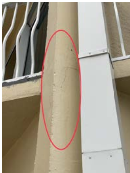
Possible concrete spalling on exterior wall near second balcony from right on the left side of the front elevation
