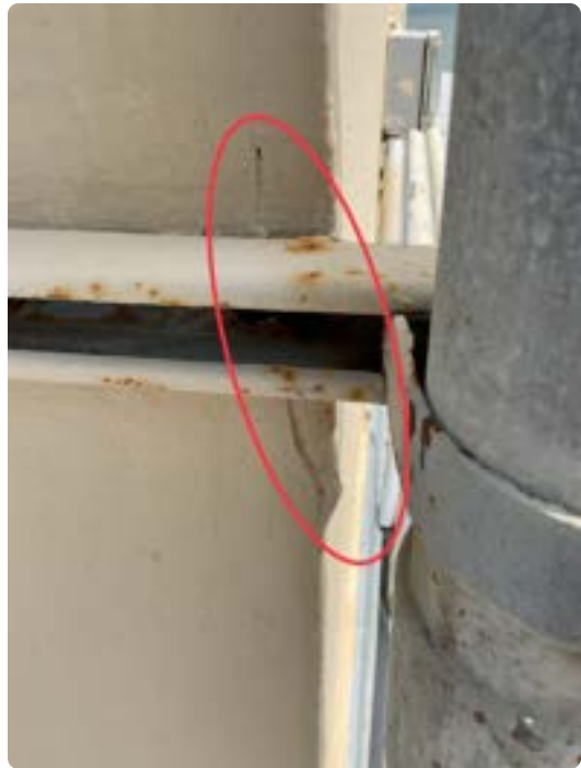
Side view of portion of concrete spalling on south exterior stairwell wall on roof
