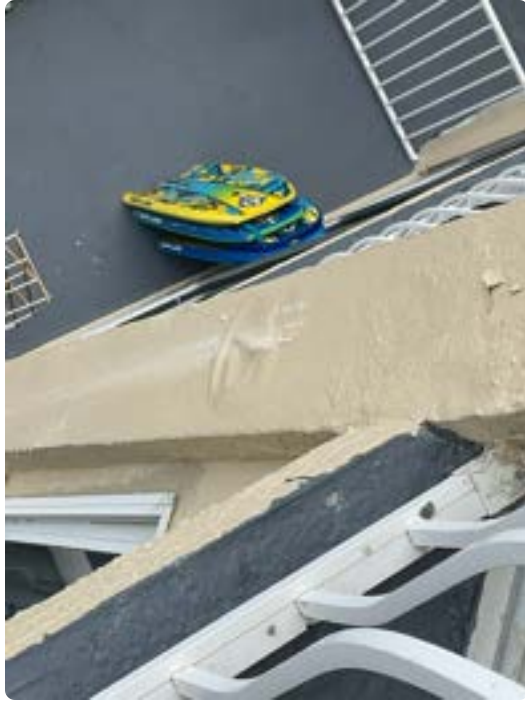
Coating bubbling on Unit 2005 balcony demising wall
