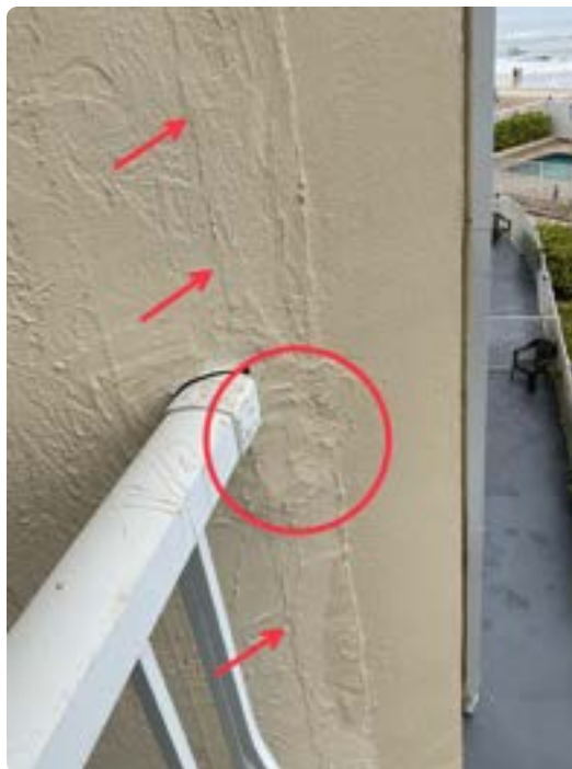
Crack in previous remediation on Unit 3004 balcony. Area is hollow where circled.
