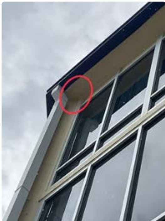
Concrete spalling in roof soffit on left side of middle of rear elevation
