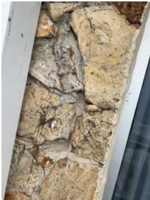
Cracks throughout stone facade grout on far-left side of rear elevation
