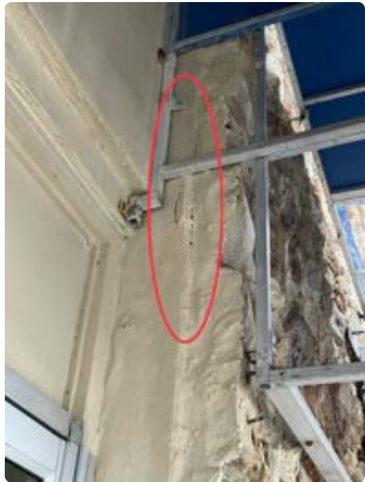
Concrete spalling on exterior wall behind stone facade on right elevation.
