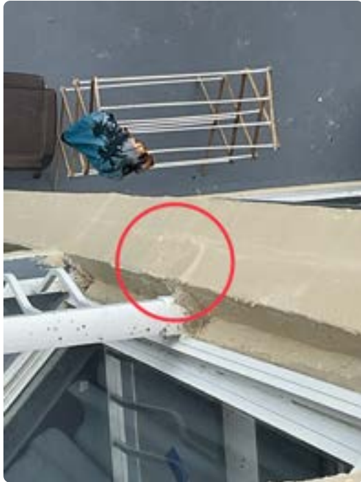
Concrete spalling near railing connection on Unit 2005 balcony
