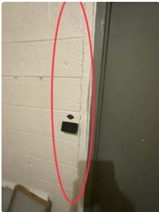
Cracked concrete to the left of roof entry door.
