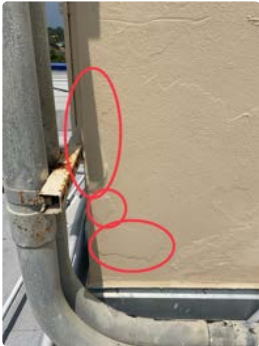
Concrete spalling on corner of southside exterior stairwell wall on roof
